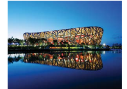
■ National Stadium (Bird's Nest)—Flame-resistance Cable
